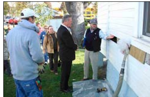
Tom Calhoun, COAD, explaining the insulation procedures to Congressman Charles Wilson
